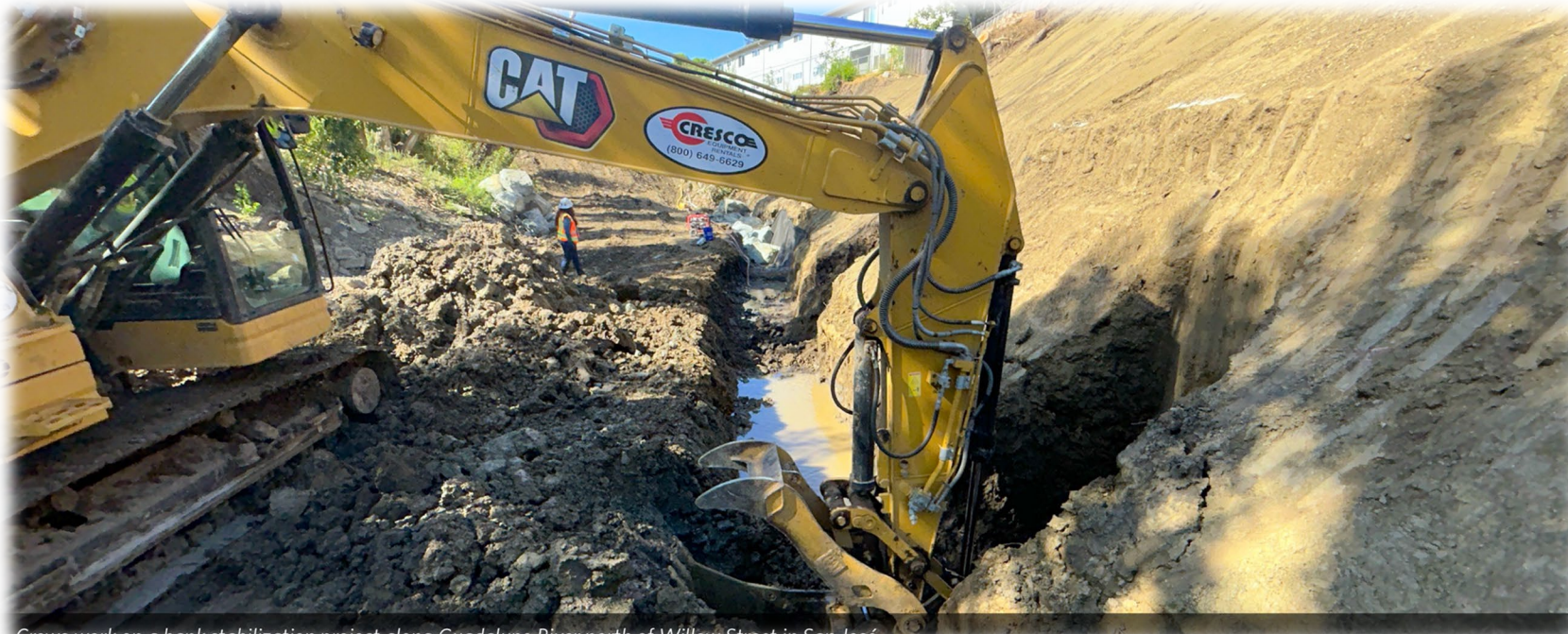
Crews work on a bank stabilization project along Guadalupe River north of Willow Street in San José.
